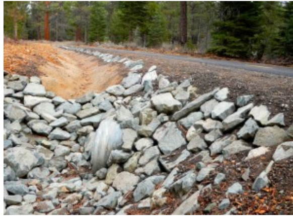
Erosion control measures line the trail.
