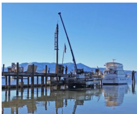
Zephyr Cove pier, where the M.S. Dixie and Bleu Wave reside, is being rebuilt. Photo Copyright 2015 Carolyn E. Wright
