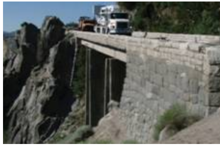
Caltrans plans to replace this Echo Summit bridge in 2019. Photo/Provided
