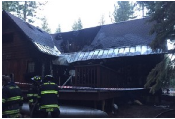
North Tahoe firefighters mop up a fire that burned the better part of a house in Tahoe City. Photo/Provided
