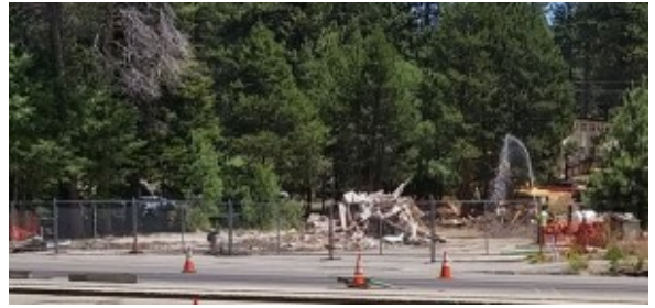
The Conservancy had the buildings razed in June 2015. Photo/Bill Kingman
