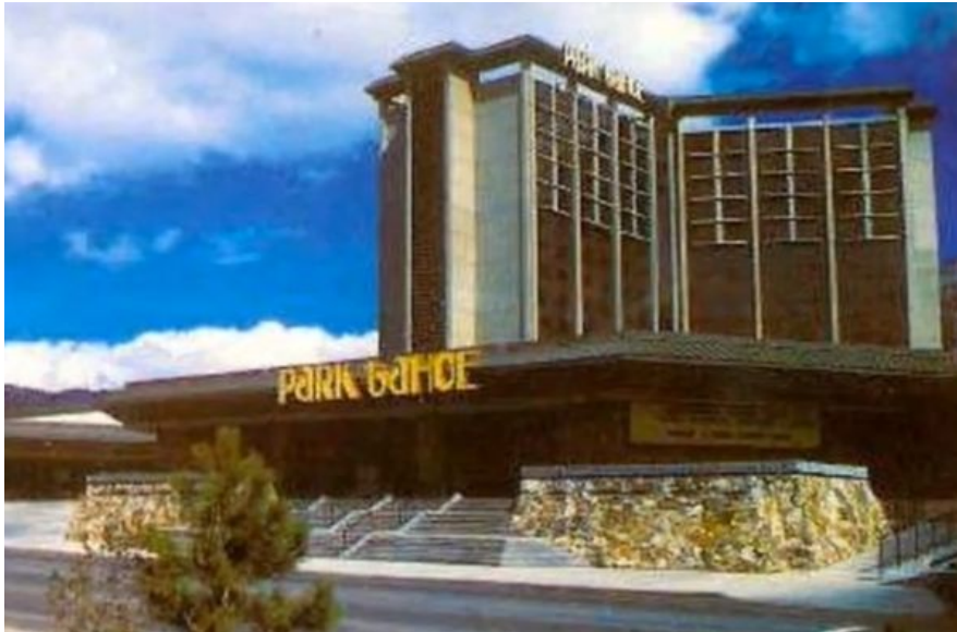
The Park Tahoe had issues at the beginning. Photo/Bill Kingman collection
