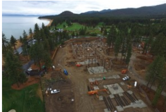
The $100 million Lodge at Edgewood Tahoe expects to be open in summer 2017. Photo/Edgewood Tahoe
