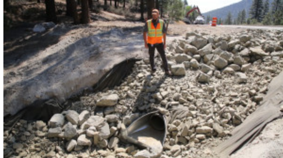
Storm drain improvements on Highway 50. Photo/Provided
