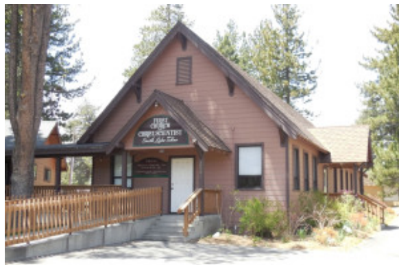
A reading room was added at left, and South Lake Tahoe Fire Station No. 3 is just to the right. Photo/Bill Kingman
