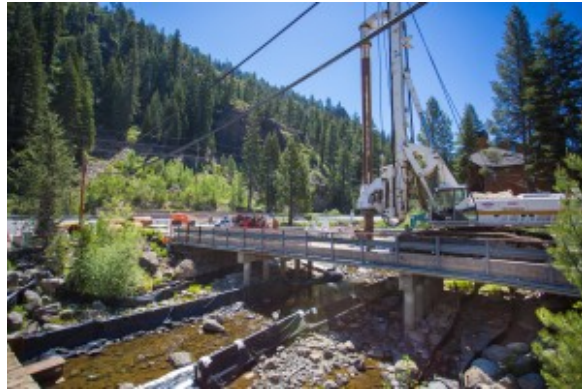
Alpine Meadows Bridge replacement. Photo/Erik Bergen
