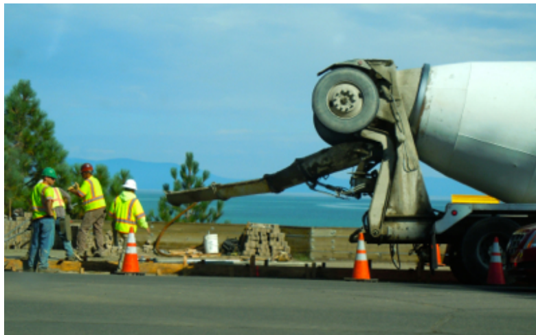
Work on Highway 50 in South Lake Tahoe will continue through at least 2019. Photo/LTN file
