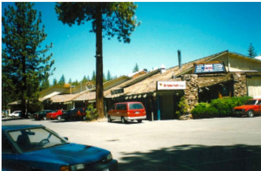
This is what the strip mall looked like 20 years ago. Photo/TRPA
