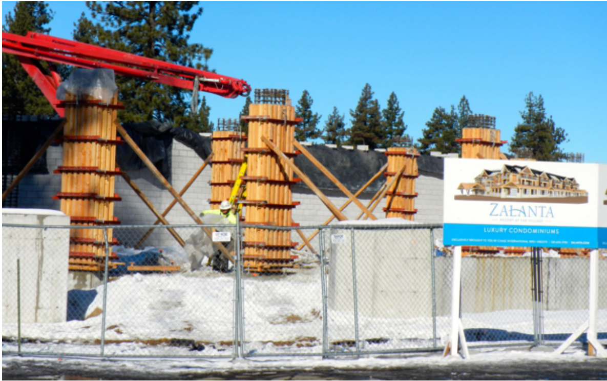
Zalanta in South Lake Tahoe will be a hotel-condo project with 32 units coming online in 2017. Photo/Kathryn Reed
