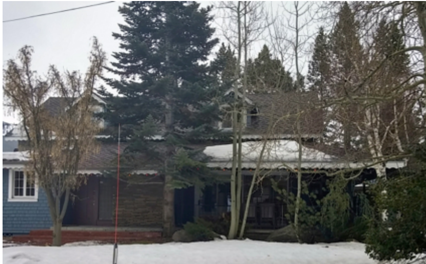
The one-time commercial building is now a private residence. Photo/Bill Kingman
