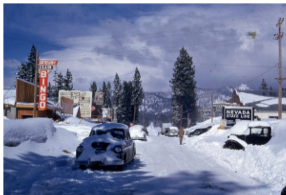
A plowed Highway 50 in 1952 allowed barely one lane of traffic. Photo/Del Laine Collection/Lake Tahoe Historical Society
