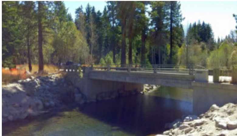
The Highway 89 bridge and Taylor Creek as viewed this month from the adjacent bicycle-pedestrian crossing. Photo/Bill Kingman
