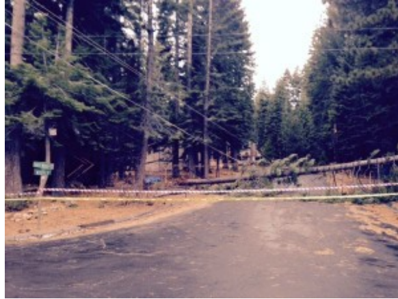
Downed power lines Dec. 11 on the South Shore. Photo/Provided
