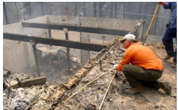
District crews crimp water supply lines in the burn area.
